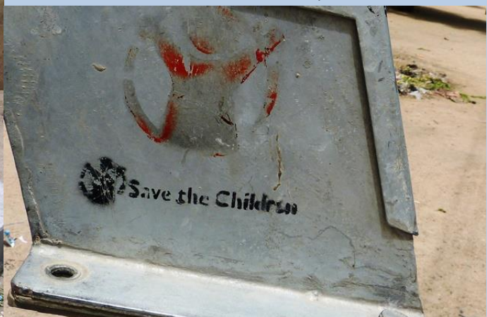
Dry hand pump and missing connexions (bolt & nuts)
