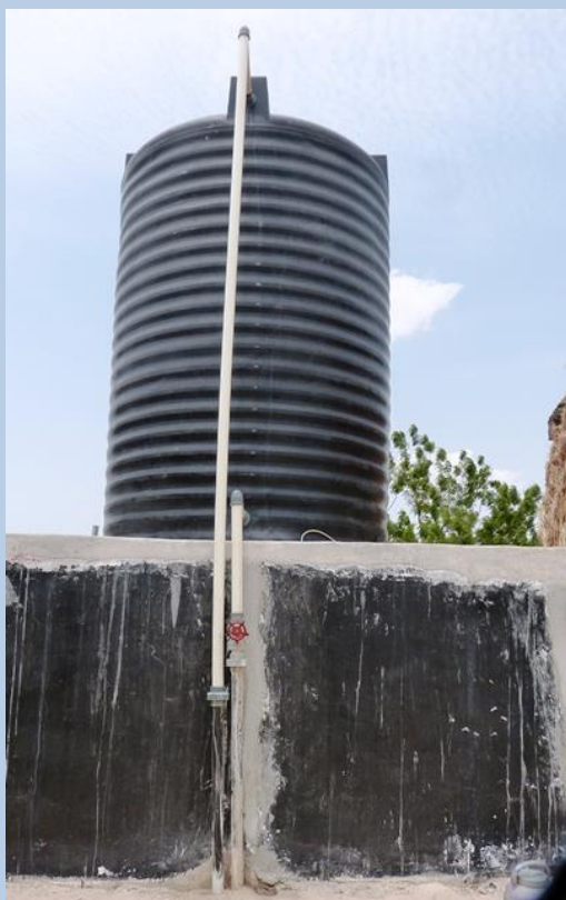
Left: 5 m3 reservoir in Alima's Clinic set by Solidarités, 50% used due to the poor performance of the NRC water network it is connected to.
