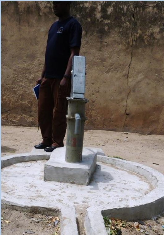
Unaligned hand pump with the upper structure slope
