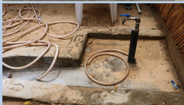
Right: Inner water network in Alina's clinic set by Solidarités: a washing equipped with two taps (up) and a single line shared by the rest of the services of the clinic. No water was available from the network at the time of the visit.
