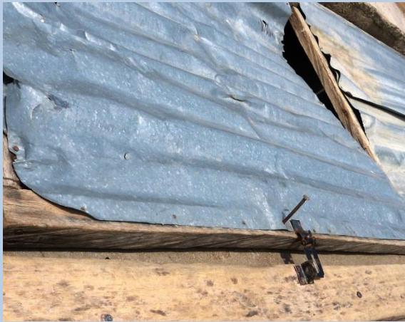
Goni Kachallari Half buried tank unprotected lid
