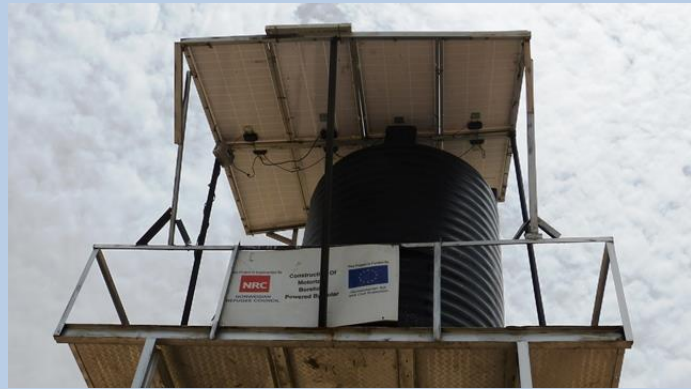
NRC solar panel array reported to have been fixed by NRC. The arrays alignment is not respected limiting energy production.
