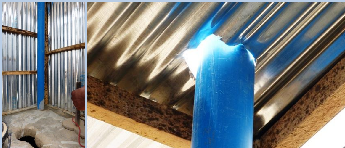
Improper ventilation pipe setting design
