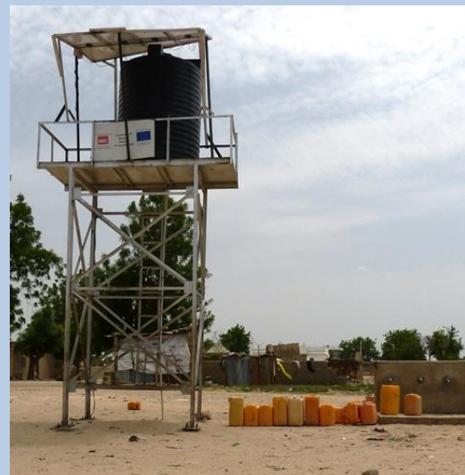
NRC water tower with damaged solar panel frame at the top of the 5 m 3 reservoir
