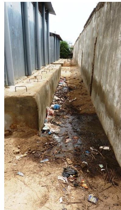
Recently “rehabilitated” latrines under UNICEF supervision in Custom House IDPs camp B with presence of open defecation creating a contamination hazard
