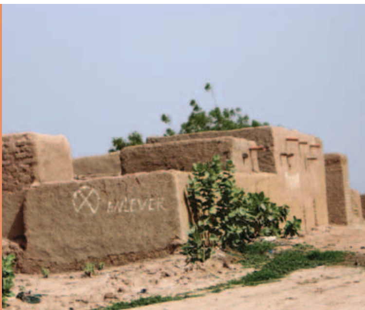
House that has to give way to an investor's project, so far without compensation for the residents
