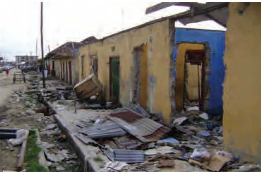
Pikine, Dakar; houses of residents being destroyed
