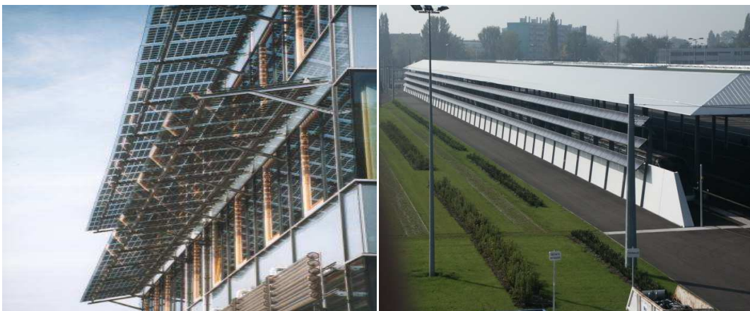
Figure 34. Perspective of existing state of the art fixed BIPV shading devices
