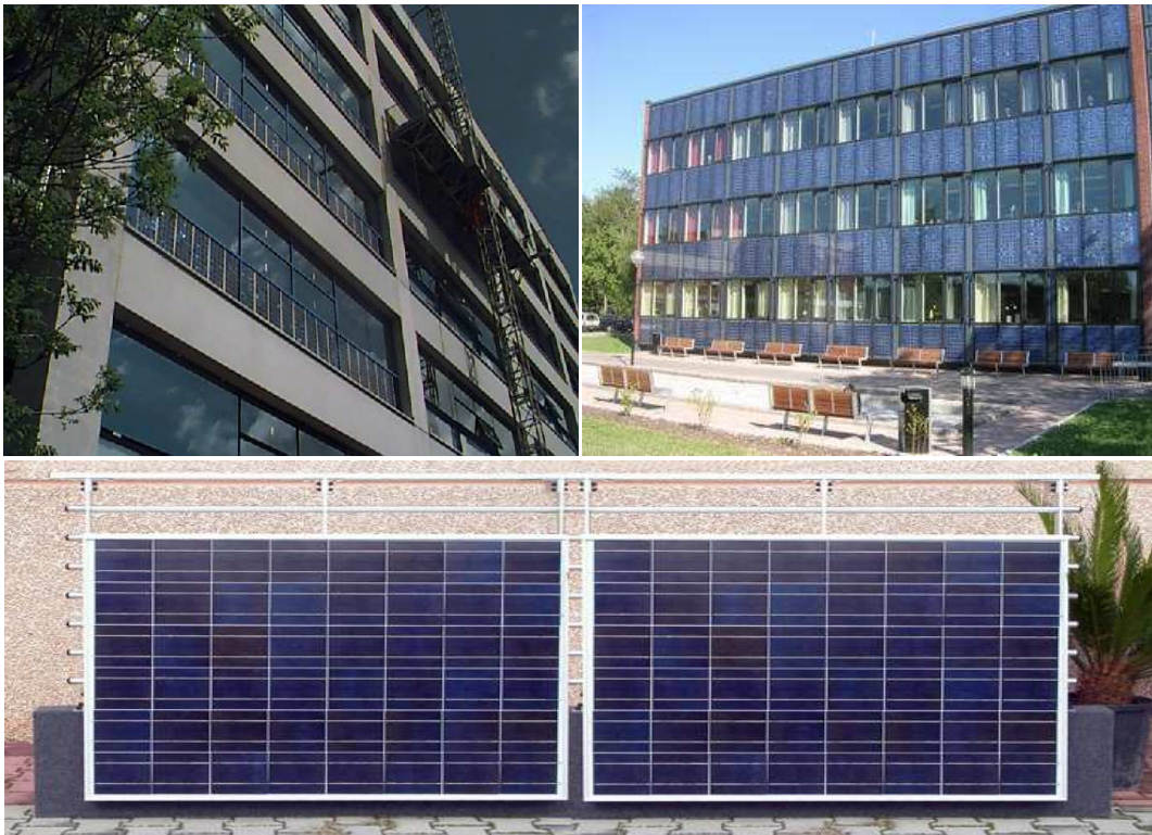
Figure 33. Perspective of existing state of the art cladding BIPV systems and opaque PV parapets (PV database - Urban Scale Photovoltaic Systems)
