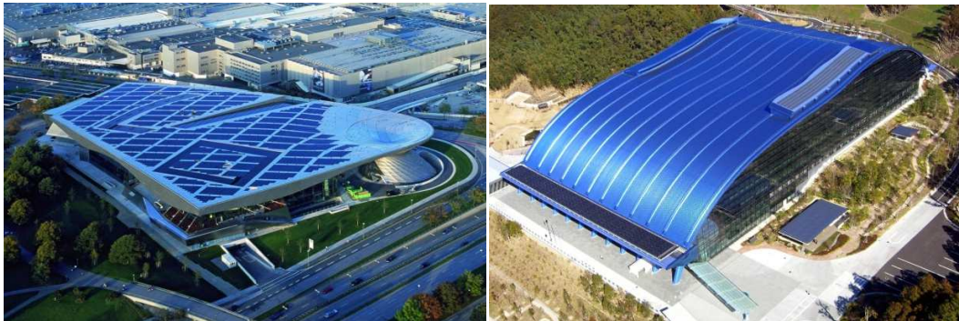
Figure 28. Perspective of existing state of the art flat and curved roof BIPV systems
