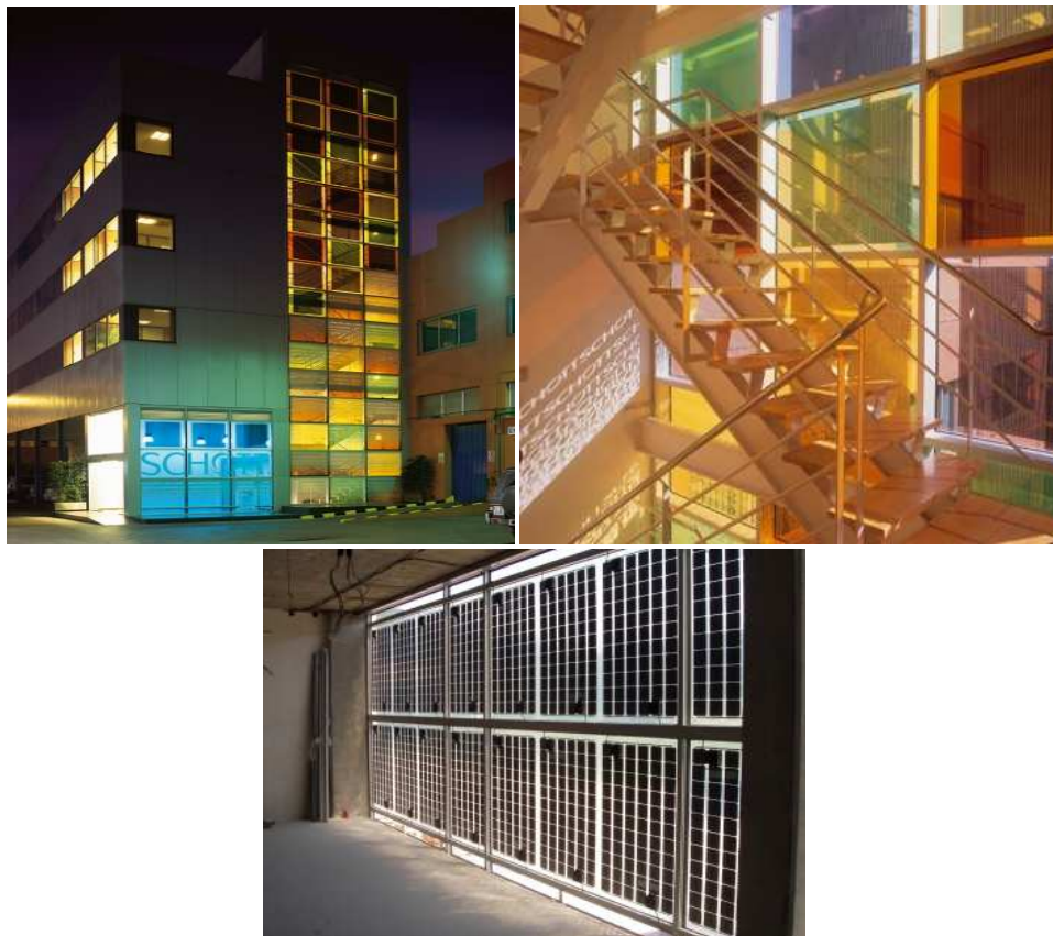
Figure 31. Perspective of existing state of the art curtain wall glazing systems with semi-transparent modules
