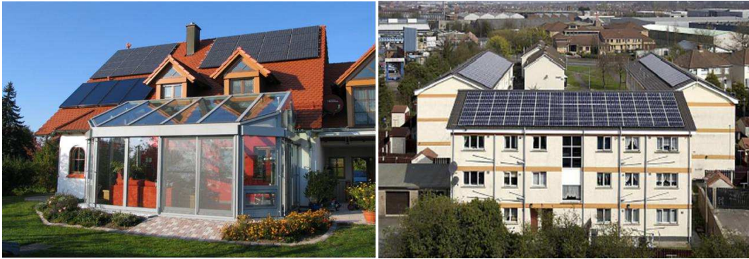
Figure 26. Perspective of existing state of the art PV installations mounted on pitched roofs
