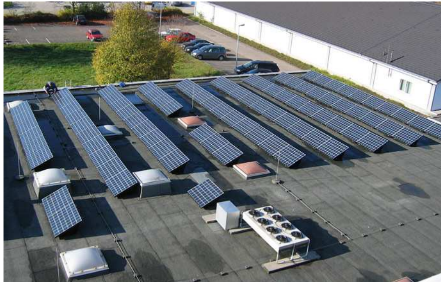
Figure 80. Example of PV arrays positioned on a flat roof with the appropriate distance between them, in order to eliminate mutual shadings
