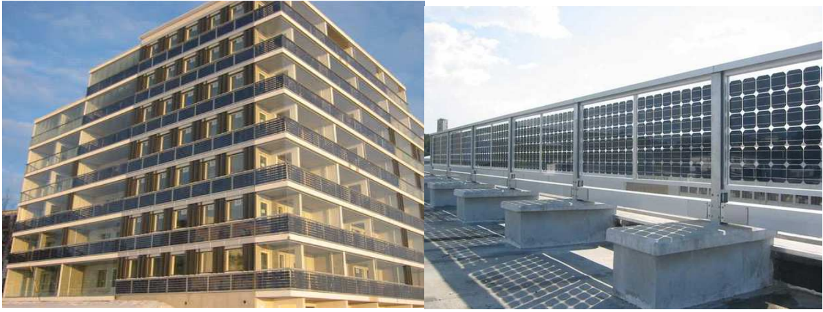
Figure 32. Perspective of existing state of the art PV parapets with semi-transparent PVs
