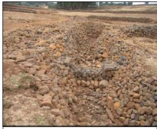
Gully treatment using check dams and Gabion in Hamusit PA
