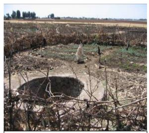
Akate PA: Shallow well constructed by the project for small scale irrigation purpose
