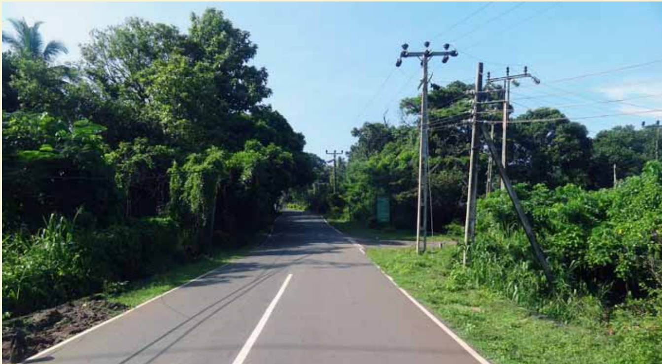
Newly constructed road at Pallekelle Industrial Estate. No potholes!
