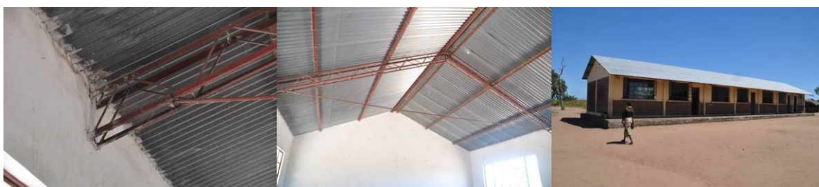
Figure 12 – School with metallic structure roof (EPC 25 de Junho – Caia District)
