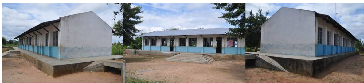
Figure 10 – EP1 Esperança Berta Sove (Chibabava District) built above a platform
