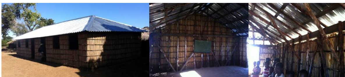
Figure 13 – School resistant to strong winds in Chinde District, Zambezia Province. Structure reinforced with “diagonais”
