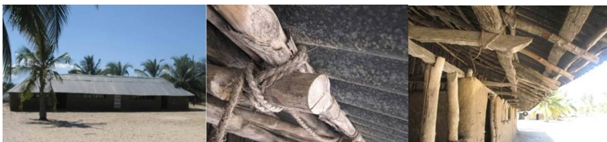
Figure 14 – Connections reinforced with local materials
