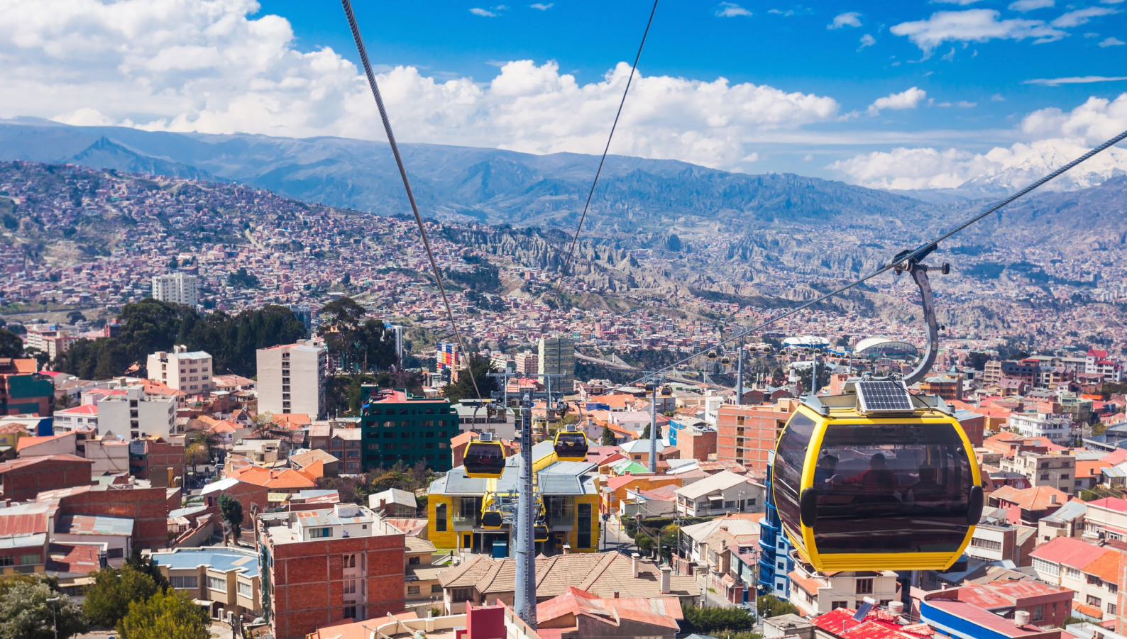
Mi Teleferico, an aerial cable car urban transit system in La Paz, is the world's highest cable car network.
